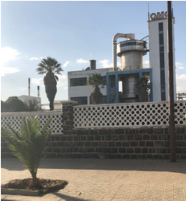
OMO factory, Asmara. Photo by Stefano Manservigi.
